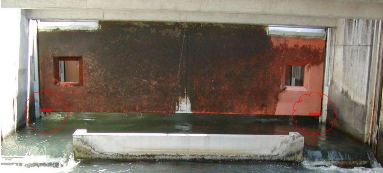
The other modifications include rounded corners within the junction pool and ladder, lamprey rest boxes on the channel floor, lamprey orifices within the fish ladder, and roughen the floors and walls in high velocity areas.
